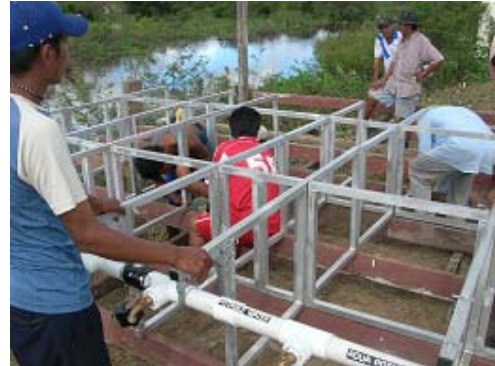
Community members assembling the support structure of the water tank.
